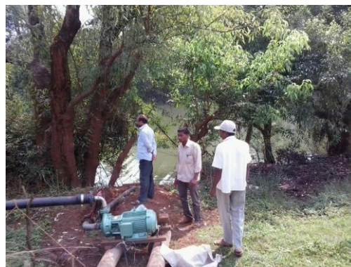
Lift Irrigation system Executed by Mahalaxmi Cluster from Kasari River For 17.90 Ha.
