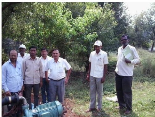
Lift Irrigation system Executed by Haritkranti Cluster from Kasari River For 11.10 Ha.
